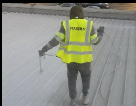
Spraying Topcoat
