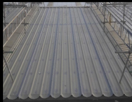
Side Lap Encapsulation
