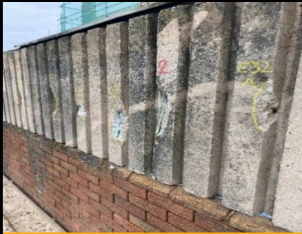
Marking up the extent of repair
