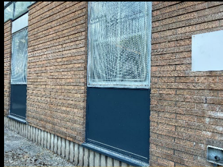
New window panels installed
