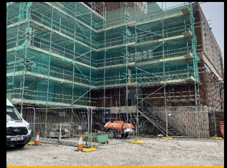
Scaffold being erected
