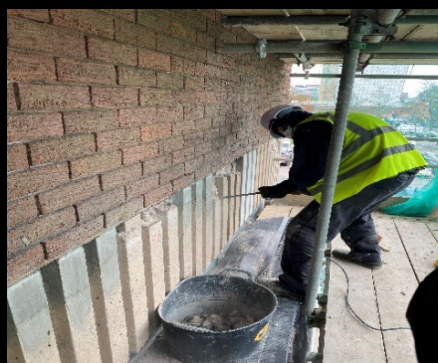
Removal of concrete
