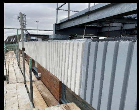
Protective coatings applied
