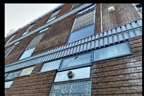
Elevation now complete
