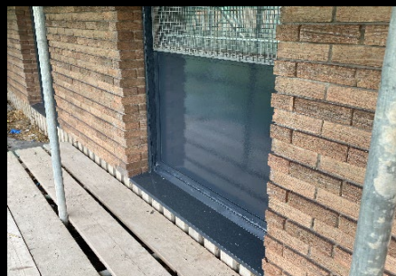
Final coat applied to panels
