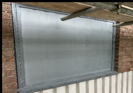
Primer coat applied to panels
