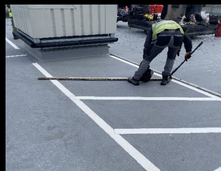
Line marking being applied
