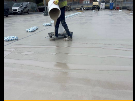
Anti-skid wearing layer applied
