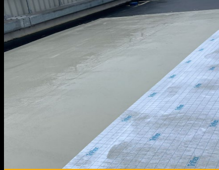
Fleece reinforcement installed
