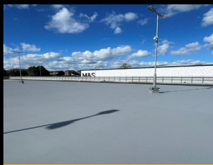
Deck coatings complete
