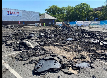
Removal of the existing tarmac
