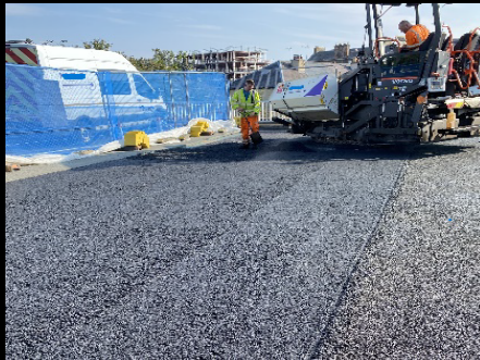
Tarmac being laid
