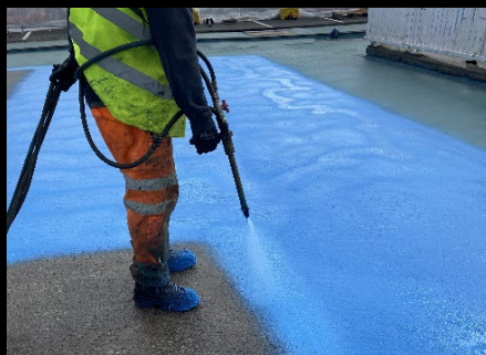
Spray applied membrane
