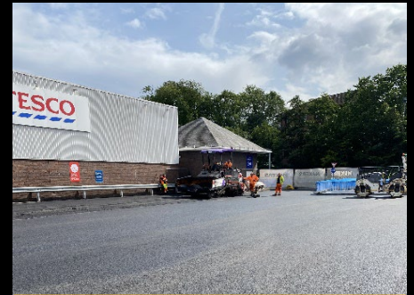
Tarmac works complete
