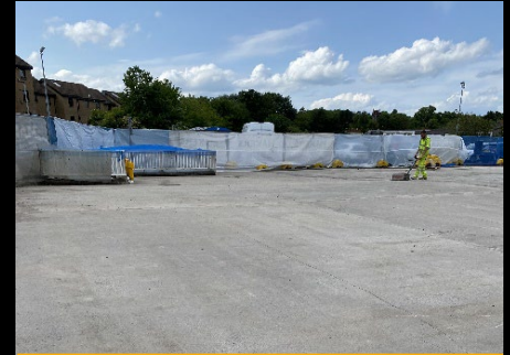
Deck prepped ready for coatings
