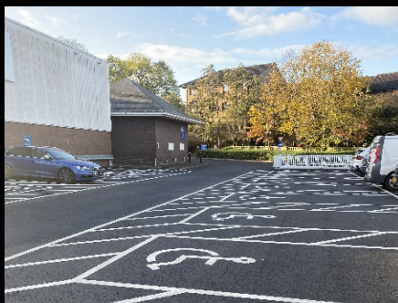
White lining completed
