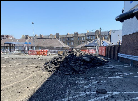
Prep works ongoing
