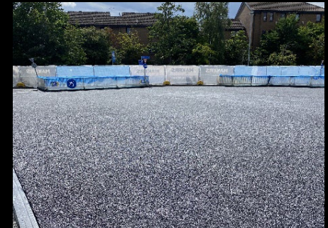
Bitumen coating fully applied
