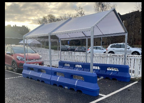
New self-weighted trolley bays
