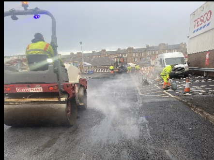
Roller compacting the tarmac
