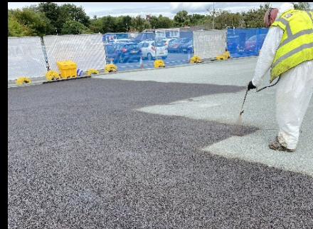
Spray applied bitumen coat
