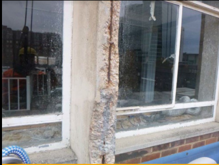
Concrete Spalls
