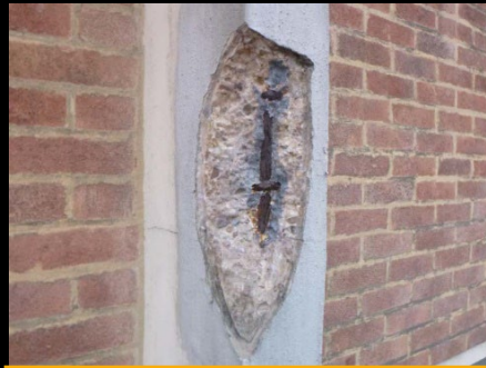
Exposed Reinforcement
