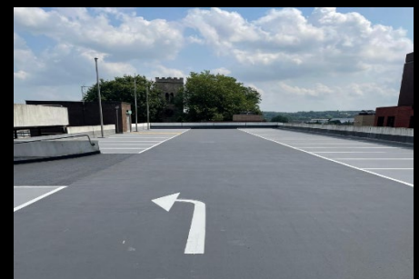
Line marking now complete
