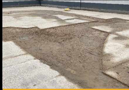
Repairs broken out
