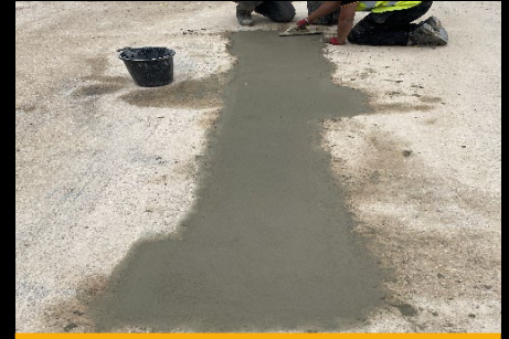
Reinstatement of repairs
