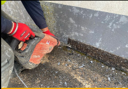
Edge prep to upstands
